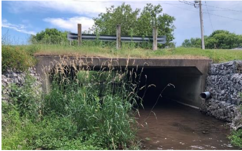
Structure 1009 on Council Road
