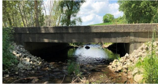
Structure 1018 on Sideroad 30
