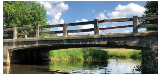
Structure 0015 on Concession 12
