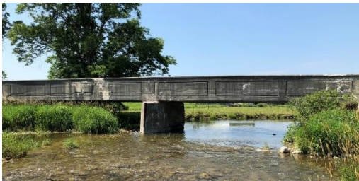
Structure 0007 on Sideroad 25N
