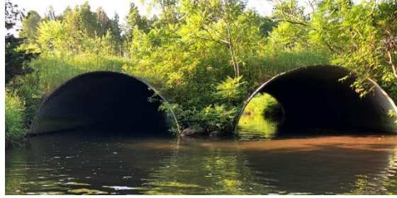
Structure 1002 on Concession 12
